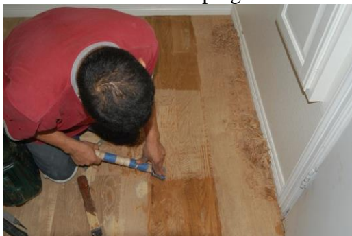
Figure 8 Scraping all dark, wet spots
